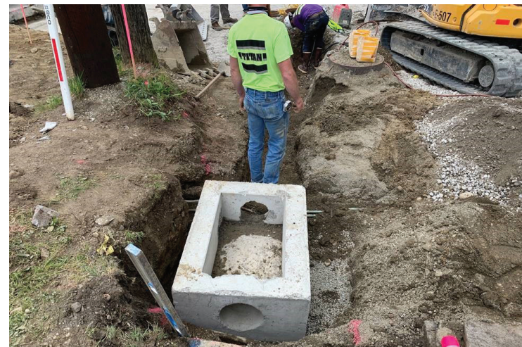
After roads and sidewalks are demolished, crews are installing drainage structures underground.
